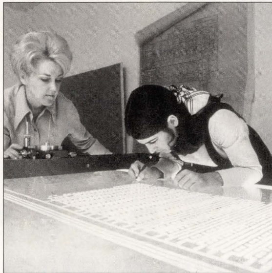
Hand-cut rubyliths were once the first step in transforming designs into hardware. As the complexity of designs increased, it became necessary to automate the drafting process, and the CAD system then replaced the X-Acto knife.
