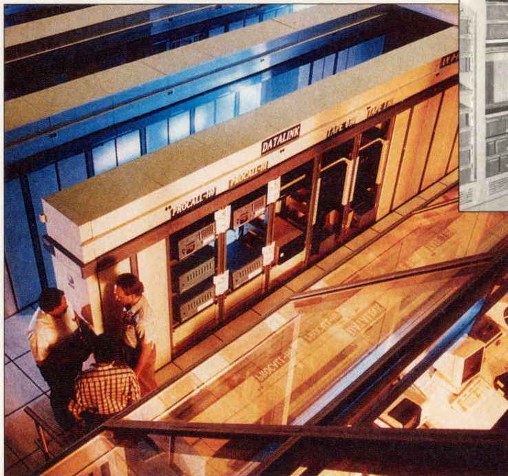
The telephone system is evolving toward digital end-to-end service, termed ISDN. Key to this transformation are switch centers tailored to a digital environment. Today's 5ESS can handle 300,000 calls per hour; 1963's ESS-1 used digital techniques to switch analog signals.
