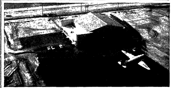
Initial unit of flight test facility
