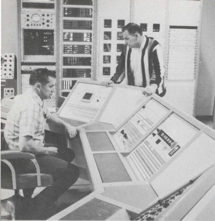
Tactical Acquisition and Data Control System being installed in the Flight Vision room tells radars where to acquire incoming planes.
