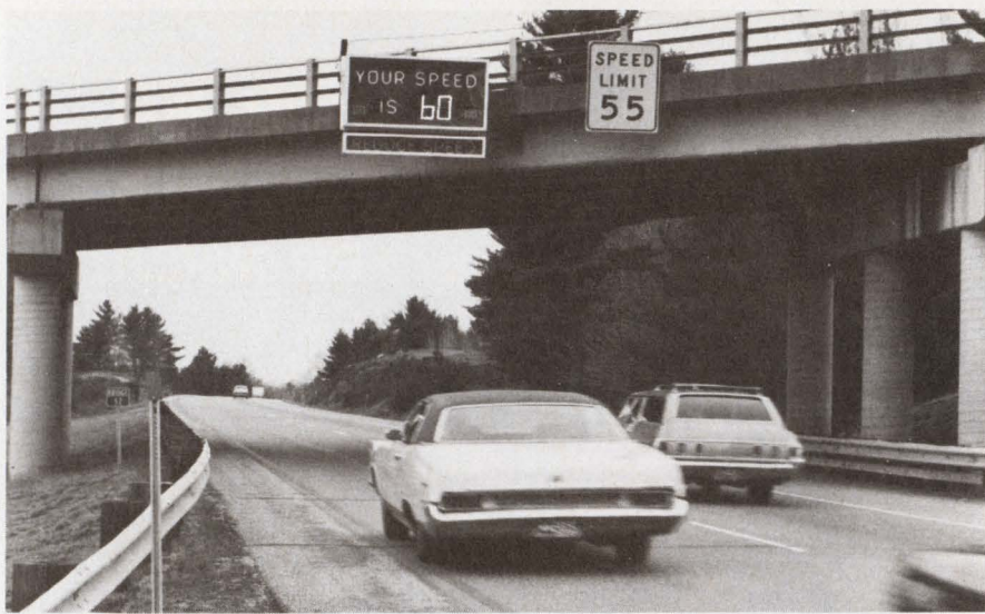
A car approaching a radar sign installed in New Hampshire is being clocked at 60 mph, five miles over the legal speed limit.
