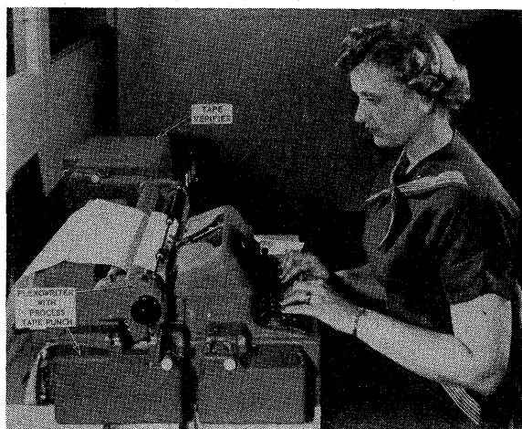
Fig. 7—Flexowriter-Verifier for preparation of process tapes.
