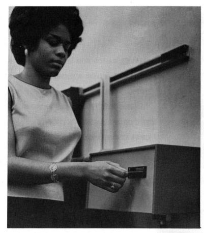
TIME RECORDING EQUIPMENT AT AMERICAN BOSCH IS CONNECTED DIRECTLY TO THE DATA PROCESSING CENTER. EMPLOYES INSERT PLASTIC CARDS INTO THE IBM 1035 DATA COLLECTION TERMINAL, AND TIME IN AND OUT IS RECORDED ON A PUNCHED CARD AT THE DATA PROCESSING CENTER.
