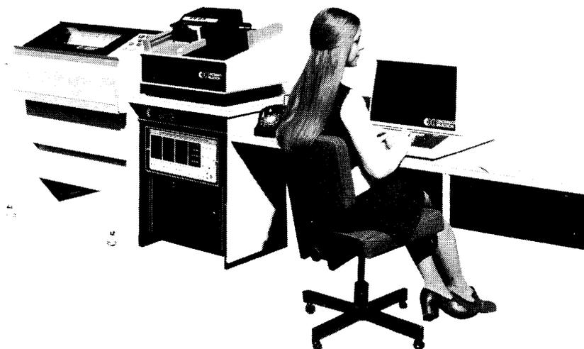
*The CIP/2200B system at left consists of a 16K-byte processor, a 600-cpm card reader, a 300-lpm printer, and a CRT console. This configuration represents the CIP/2200B being used as a remote batch terminal.*
