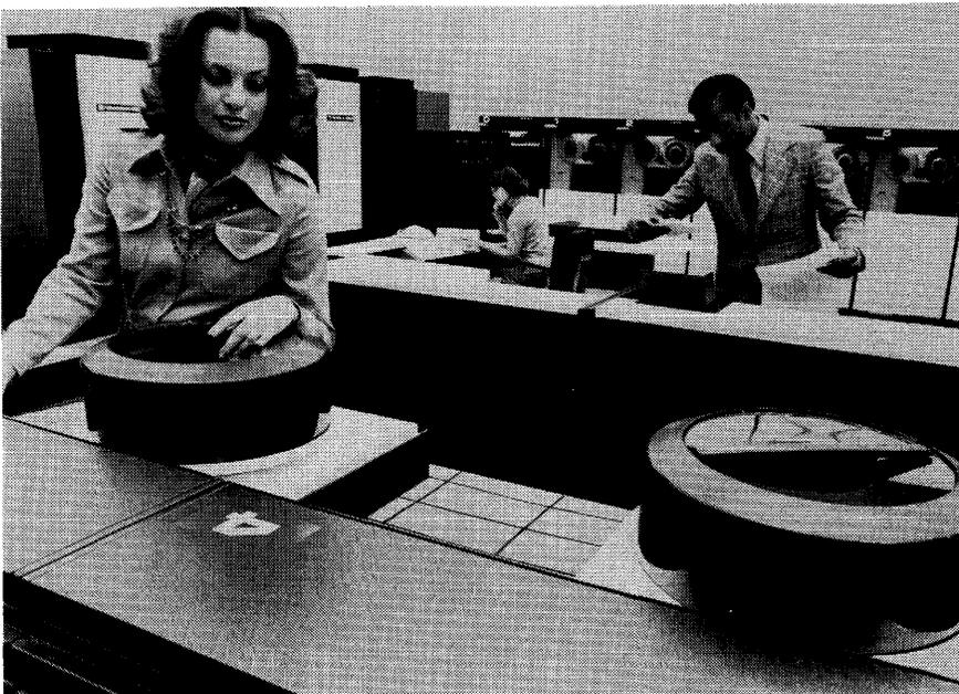
*The Model 66/80 is the most powerful of the five large-scale Level 66 processor models. The Level 66 systems are quite similar to Honeywell's successful Series 6000 computer family and offer Series 6000 users a clear upward growth path. Monthly rentals for Level 66 systems range from about \$16,000 to over \$100,000.*
