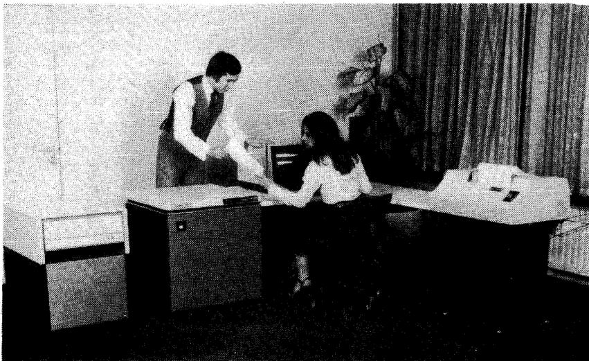
The ICL System Ten, using a hard-wired partitioning technique within the CPU to achieve multiprogramming, can concurrently process up to 20 independent jobs. The 220 Series Model 3 Entry-Level System shown here includes, from left, a Model 43 fixed/exchangeable disc drive for 8 million characters of on-line storage, a Model 22 processor with a 20,000 character memory, a Model 85 Visual Display Unit for user input and system control, and a 165-cps Model 51 serial printer.
