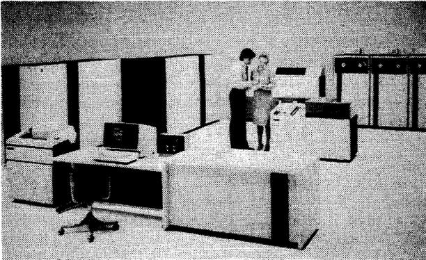
*ICL has introduced two ultra-high powered computer systems - the Atlas 10 Models 15 and 25. Both are compatible with the largest IBM and other plug-compatible computers and have processing powers between three and five times greater than the IBM 3033 computer.*
