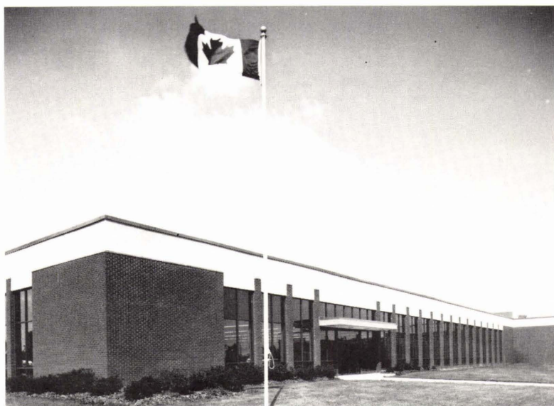
DIGITAL Facility, Kanata, Canada
